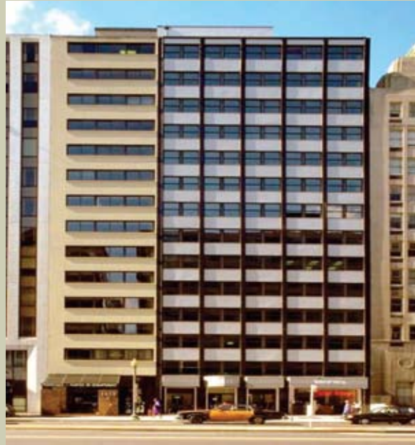
FAÇADE PRIOR TO RENOVATION
