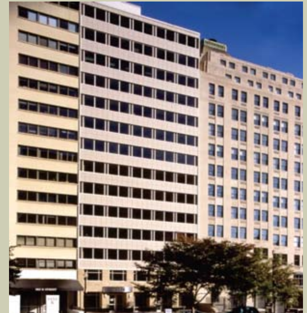
FAÇADE POST RENOVATION
